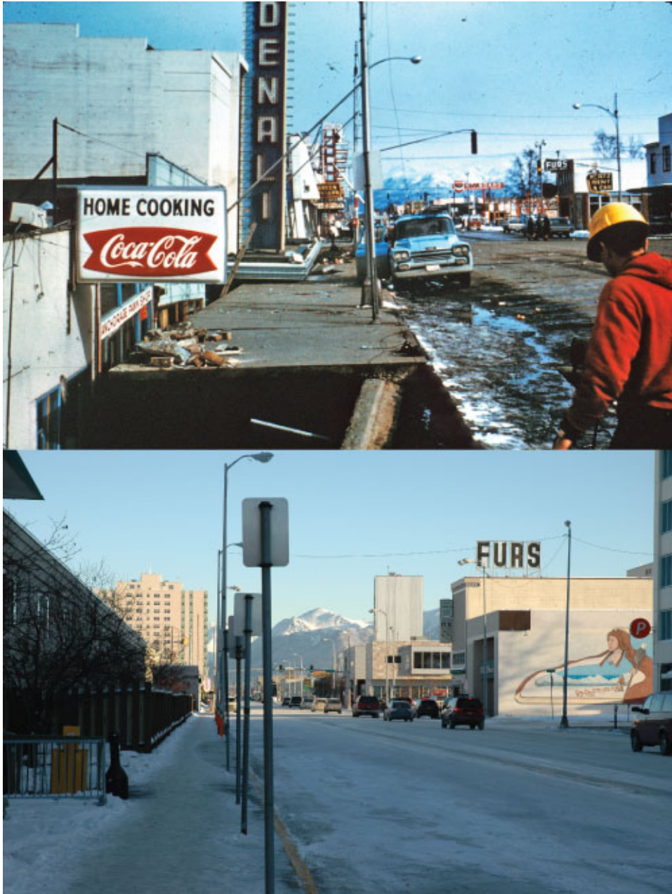
Figure 14. Comparison photographs taken from the same location on 4th Avenue about 1 block east of the main area of damage, Anchorage, Alaska. In 1964 (top), the ground just to the left of the sidewalk dropped about 8 feet bringing the marquee of the Denali Theater down to street-level. (Top photograph from U.S. Geological Survey Photographic Library, ID aeq00046, 1964; bottom photograph taken by R.G. McGimsey, U.S. Geological Survey, 2013.)
