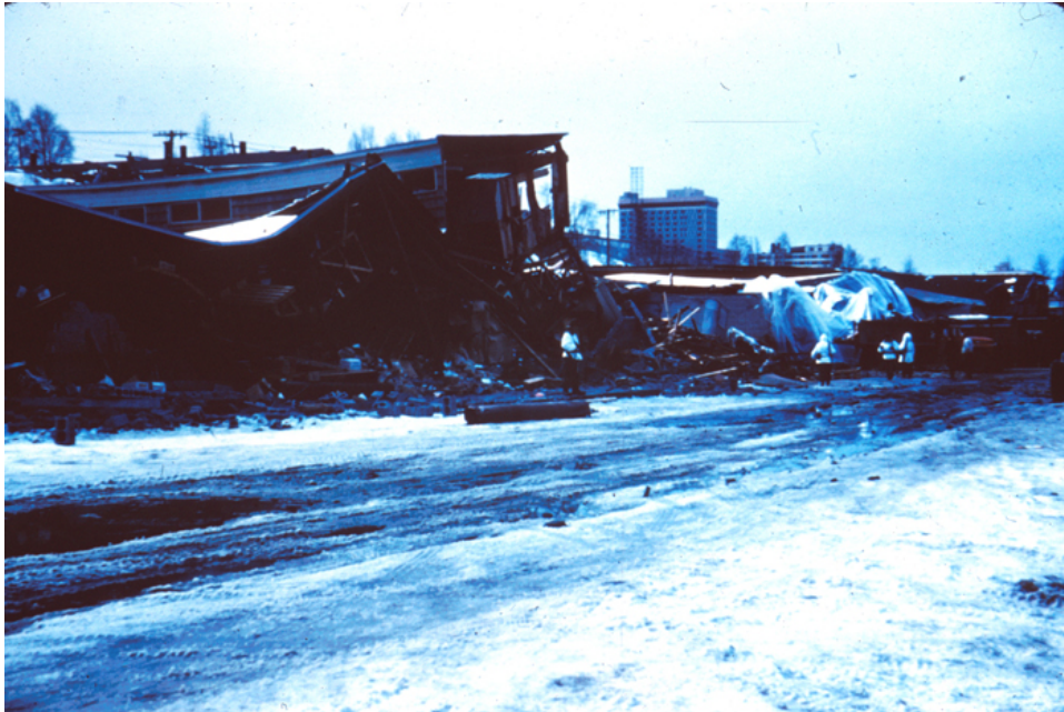
Figure 11. View looking southwest from 1st Avenue of warehouses damaged by compressional deformation at the toe of the 4th Avenue Slide, Anchorage, Alaska, 1964. The Westward Hotel (Stop 13) can be seen in the background. (Photograph from U.S. Geological Survey Photographic Library, ID aeq00051.)
