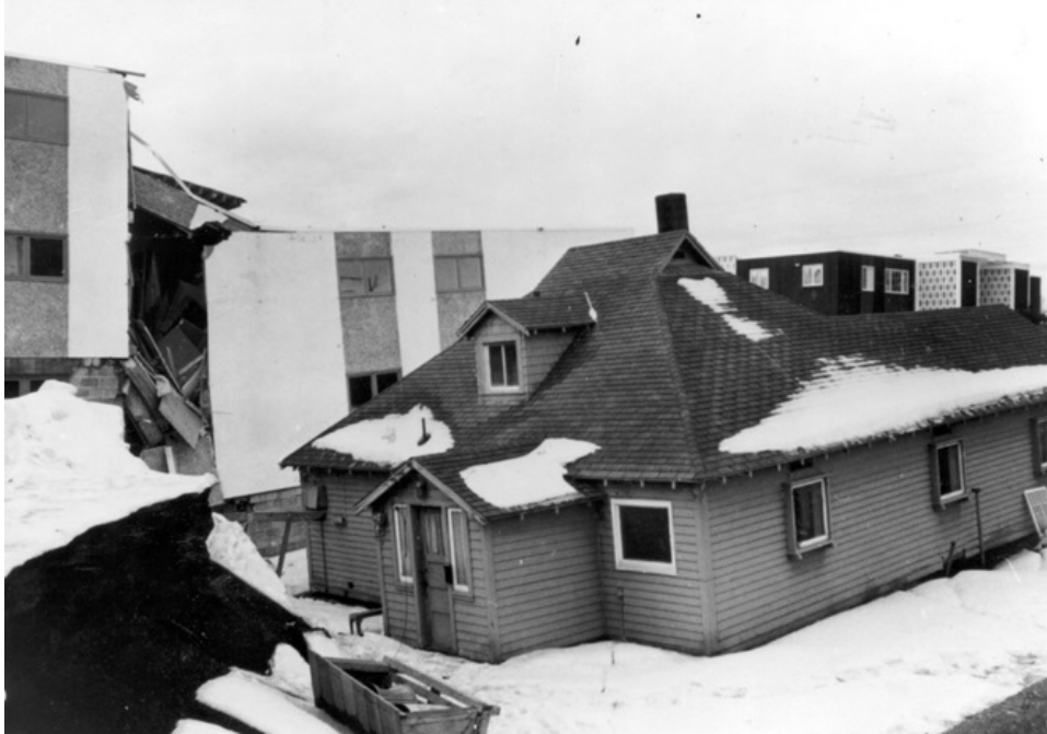
Figure 30. The apartment building behind the largely undamaged house in the foreground was sheared almost equally in two when the western half dropped 7 feet down the main scarp at the head of the L Street Slide, Anchorage, Alaska, 1964. The apartments have been removed but the Anchorage Medical and Surgical Building to the east was undamaged. (Photograph from U.S. Geological Survey Photographic Library, ID ake00327.)
