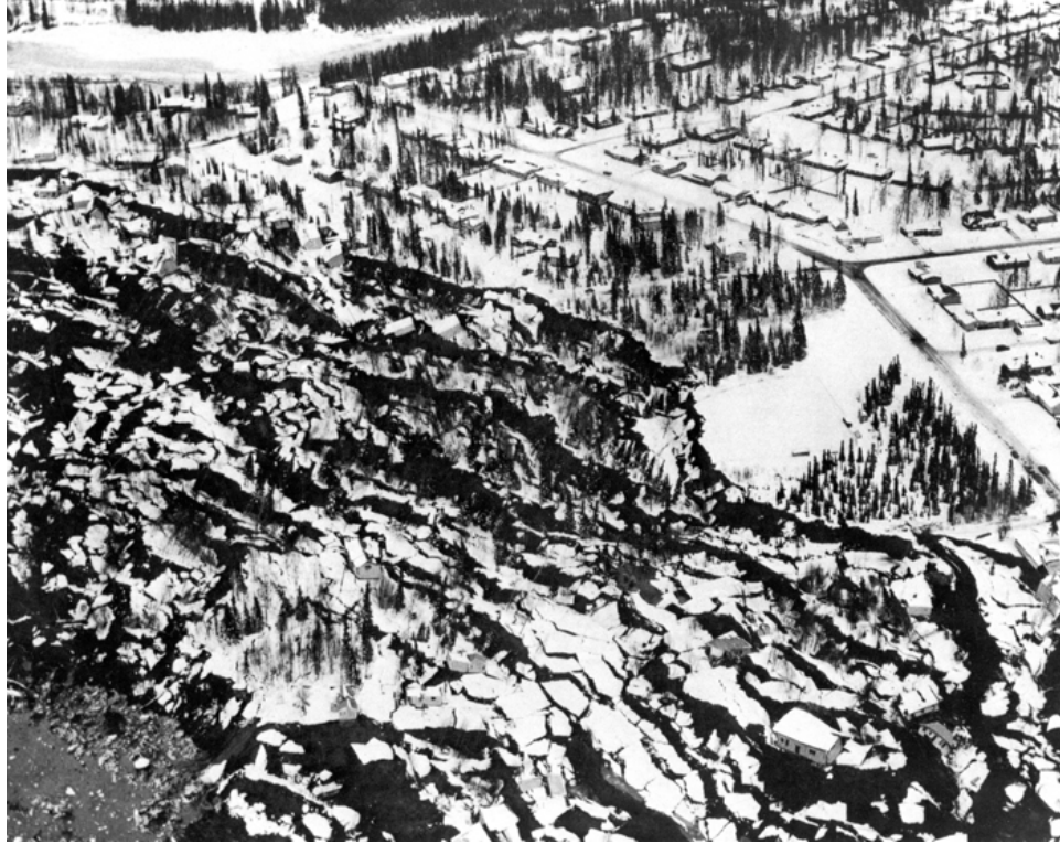
Figure 37. View of part of the Turnagain Heights Slide looking roughly southeast shortly after the earthquake, Anchorage, Alaska, 1964. (Photograph from U.S. Geological Survey Photographic Library, ID ake00087.)
