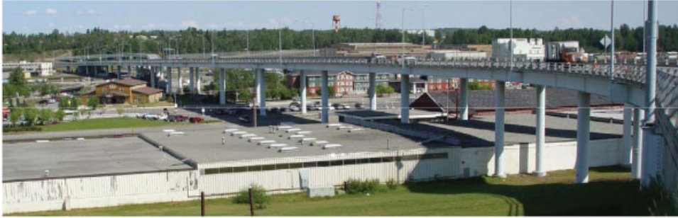
Figure 13. View looking north from Buttress Park of the Port Access Bridge (photograph from Yang, 2006, p. 4), Anchorage, Alaska. Accelerometers are installed near the tops of many of the support columns.
