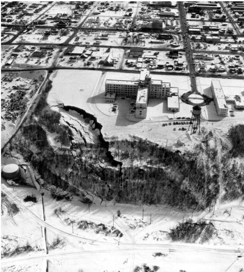
Figure 6. Oblique aerial view looking south of the Native Hospital Slide and the former Alaska Native Service Hospital, Anchorage, Alaska, 1964. The damaged fuel tank from Stop 3 (fig. 5) can be seen below the middle of the left margin of the photograph. (Photograph from U.S. Geological Survey Photographic Library, ID ake00065.)
