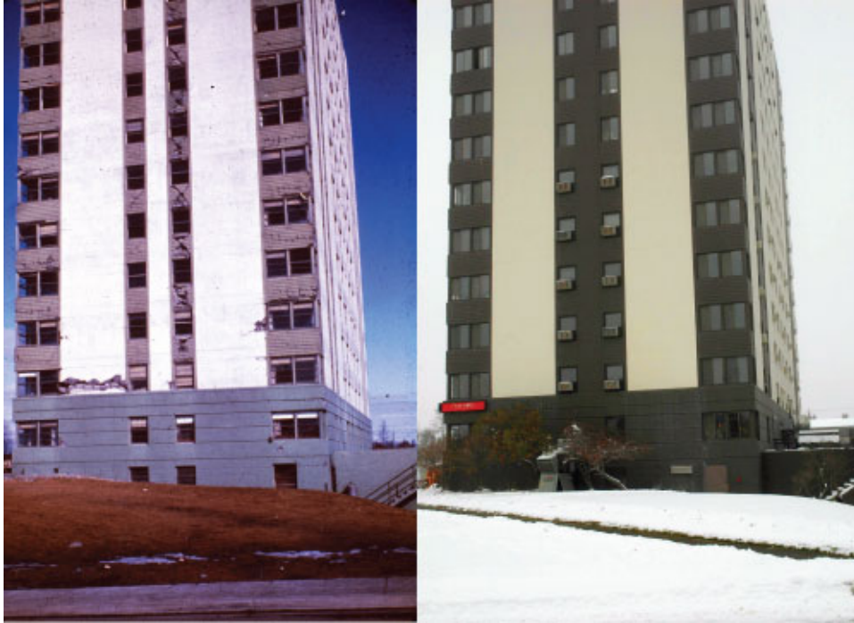
Figure 28. Comparison photographs of the Inlet Tower taken from the same location on 13th Avenue. (Left photograph [1964] from U.S. Geological Survey Photographic Library, ID aeq00019; right photograph [2013] taken by R.G. McGimsey, U. S. Geological Survey.)
