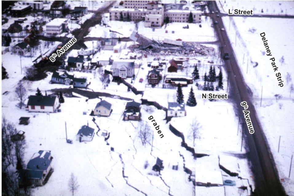
Figure 34. In this annotated view looking east, the graben at the head of the L Street Slide, Anchorage, Alaska, 1964 cuts through properties between 8th and 9th Avenues from upper left to lower right. The collapsed Four Seasons Apartment Building (Stop 23) and the relatively undamaged St. Mary's Residence (Stop 22) lie beyond the graben on undisturbed ground. The present-day Centennial Rose Garden is just off the right margin of this photograph, near the N Street easement. (Photograph from U.S. Geological Survey Photographic Library, ID aeq00043.)
