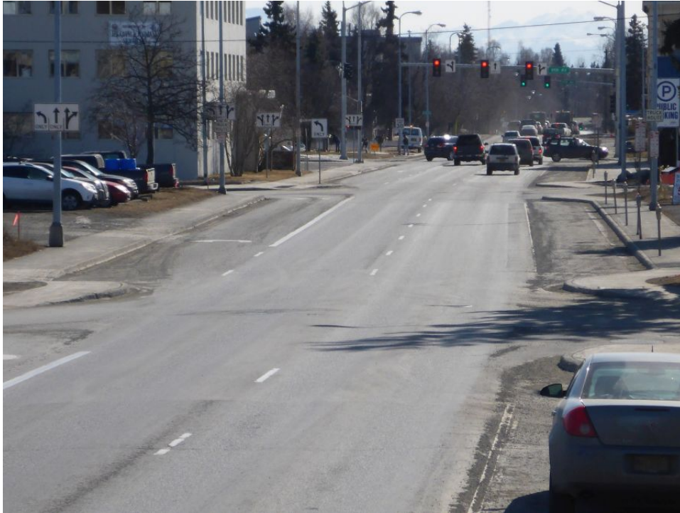
Figure 31. View looking south down L Street from a just south of 6th Avenue, Anchorage, Alaska. The two subtle but distinct kinks in the centerline, as it is traced from lower left toward the upper right, represent the re-alignment of L Street where it crossed the main scarp at the head of the L Street Slide. (Photograph taken by Evan Thoms, U.S. Geological Survey [2014].)
