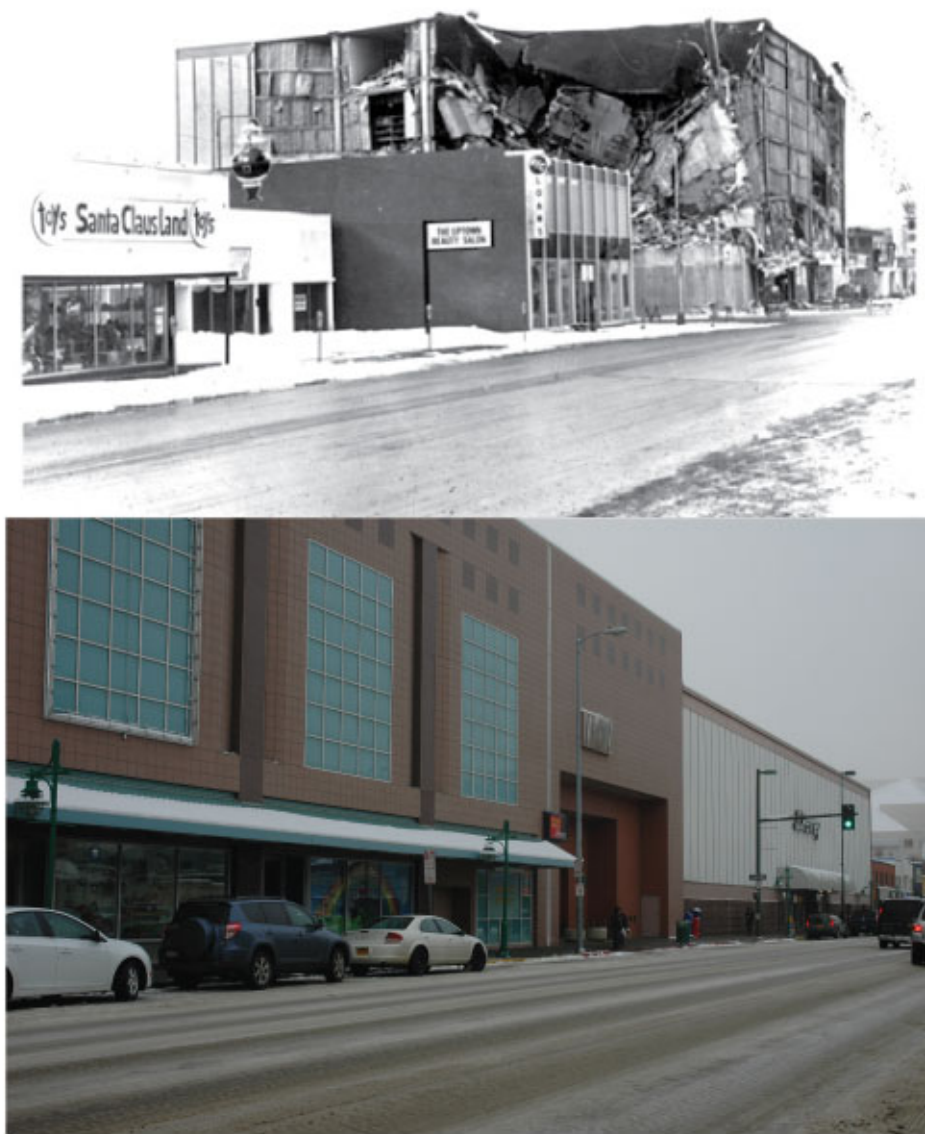
Figure 19. Comparison photographs of the J.C. Penney Building from 5th Avenue looking west, Anchorage, Alaska. (Top photograph [1964] taken by U.S. Geological Survey; bottom photograph [2013] taken by R.G. McGimsey, U.S. Geological Survey.)
