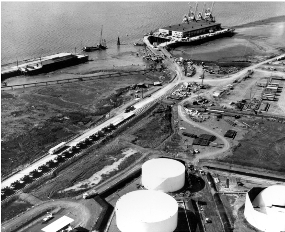
Figure 12. Anchorage municipal wharf area at low tide, shortly after the earthquake, Anchorage, Alaska, 1964. The main dock was slightly damaged, but the older U.S. Army dock (upper left) was ruined. Vibration and ground fractures damaged some structures in the port area, including the fuel tank seen in the lower right. (Photograph from U.S. Geological Survey Photographic Library, ID ake00243.)
