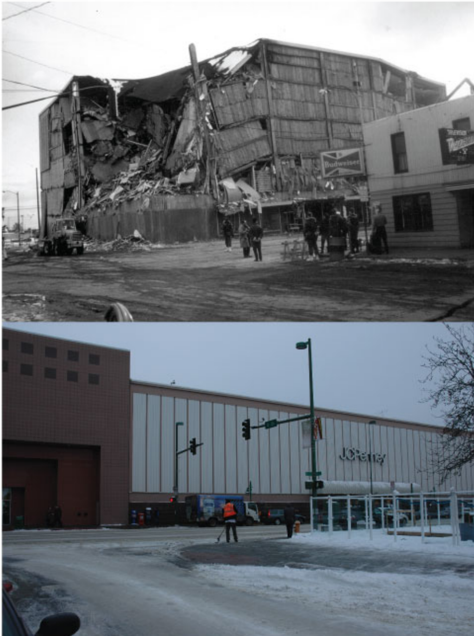
Figure 18. Comparison photographs of the J.C. Penney Building from D Street looking southwest, Anchorage, Alaska. (Top photograph [1964] taken by George Plafker, U.S. Geological Survey Photographic Library, ID ake00055; bottom photograph [2013] taken by R.G. McGimsey, U.S. Geological Survey.)
