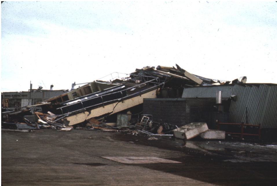
Figure 42. The destroyed control tower at the Anchorage International Airport, Anchorage, Alaska, 1964. (Photograph from U.S. Geological Survey Photographic Library, ID aeq00027.)
