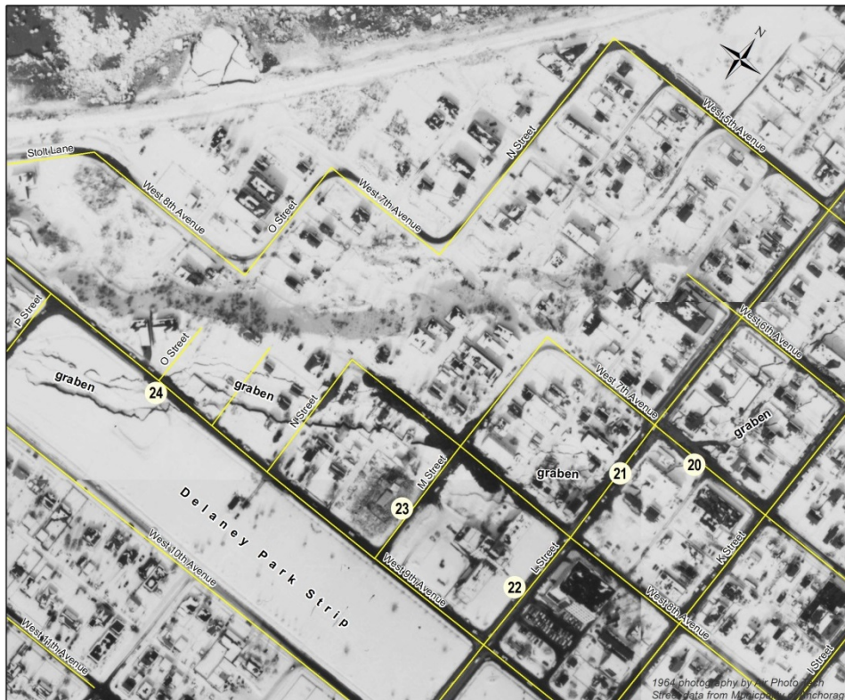
Figure 29. Annotated aerial photograph of most of the area affected by the L Street Slide, Anchorage, Alaska. Photographic tour stops are marked by number: (20) 715 L Street Apartment Building, (21) L Street Bend, (22) St. Mary's Residence, (23) Four Seasons Apartment Building, and (24) L Street Slide scarp. (Photograph taken by Air Photo Tech, 1964.)
