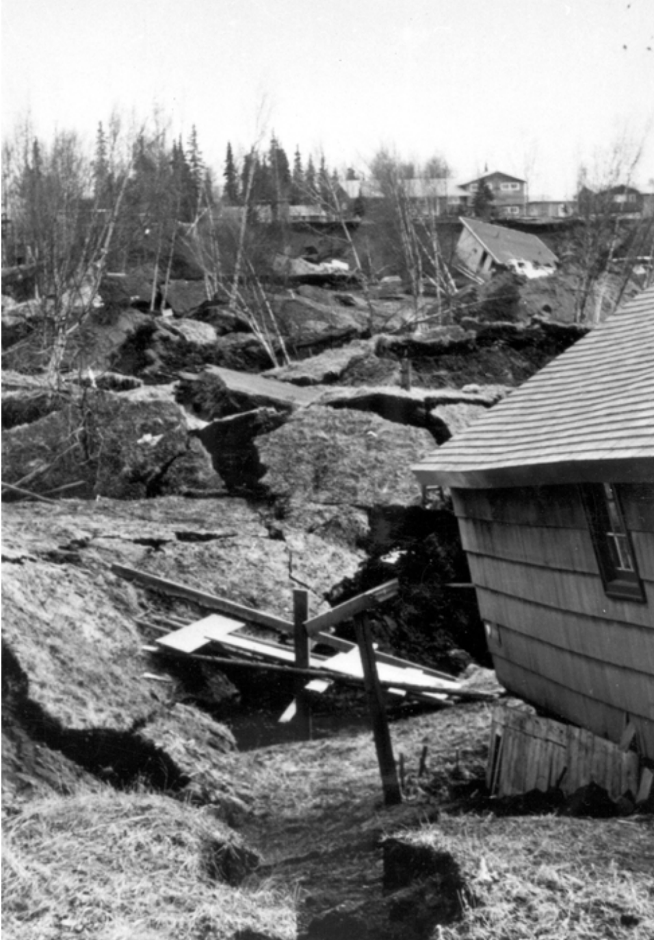
Figure 38. View from within the Turnagain Heights Slide mass looking roughly south, Anchorage, Alaska, 1964. Note the structures on the new bluff in the background. The ground surface was lowered about 35 feet from the pre-quake level. After the earthquake this area was regraded and gradually redeveloped with single-family residences. (Photograph from U.S. Geological Survey Photographic Library, ID eib00337.)
