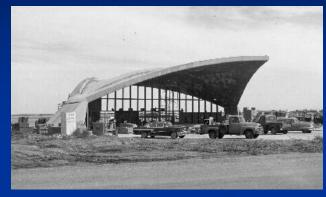
Candela has taken the simple geometric shape of the HP shell and used it to introduce a dazzling array of variations into architecture. All of his works, including this enormous 60m X 90m space, are constructed in four centimeter thick reinforced concrete. When asked how he manages to make it so thin, he says enthusiastically...
